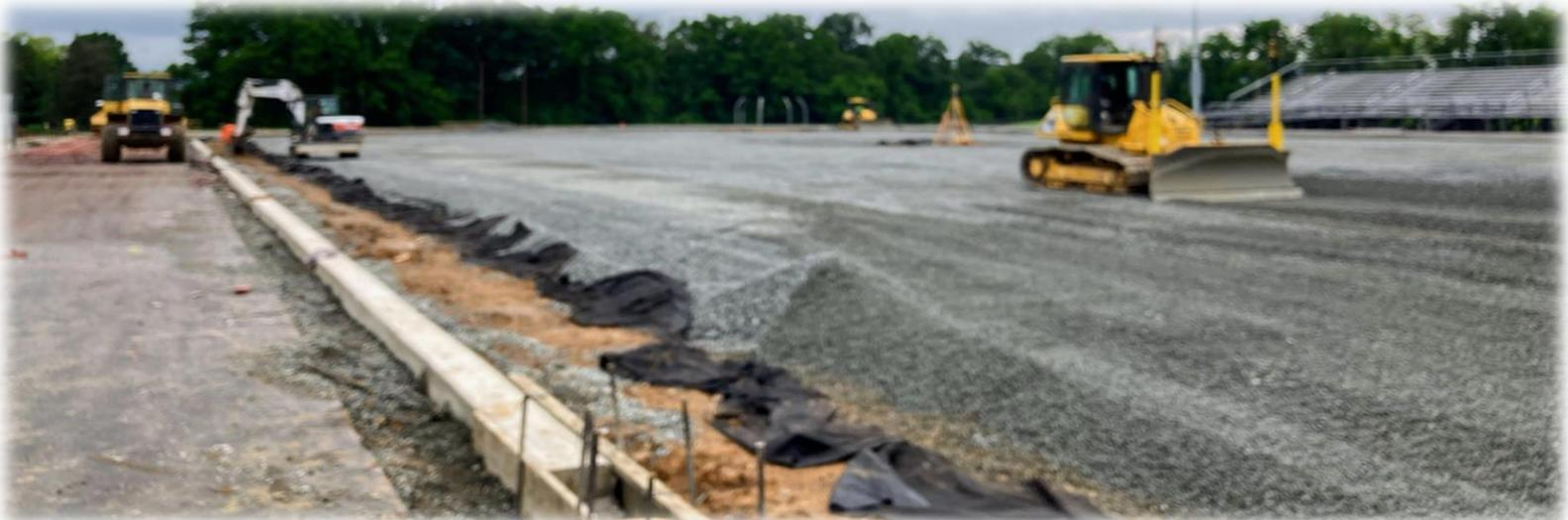
Figure 1 Synthetic Turf Sub Base preparation to ensure a flat/planar surface that will stay that way over the entire field, as well as ensuring proper long term drainage.
