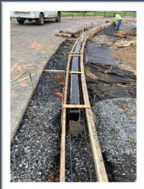
Figure 2 On the Left shows design detail of drainage to capture run off from track surface with installation of ACO approved drainage system.
